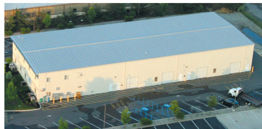
Farmingdale, NJ facility
