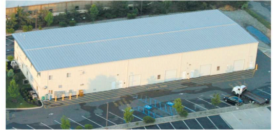
Farmingdale, NJ facility
